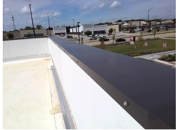
Parapet Wall Panera, Smashburger:
