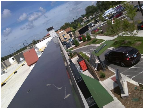
Parapet Wall Panera, Smashburger:
