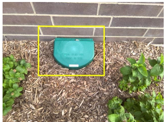
LANDSCAPING/RODENT TRAPS/EXPOSED WIRES: Right side smash burger
