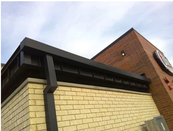
Roof Drainage System Canes:
