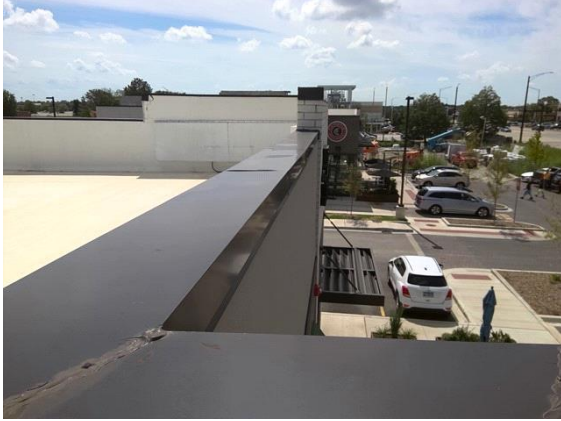
Parapet Wall Panera, Smashburger:
