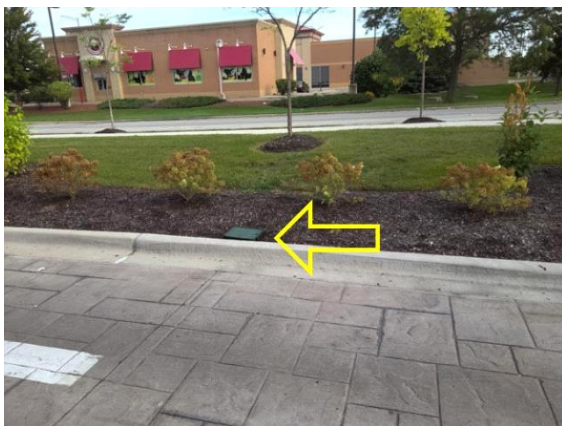
LANDSCAPING/RODENT TRAPS/EXPOSED WIRES:
