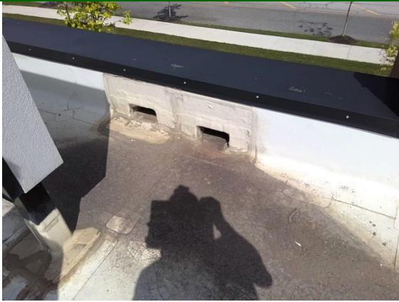
Roof Drainage System Canes:
