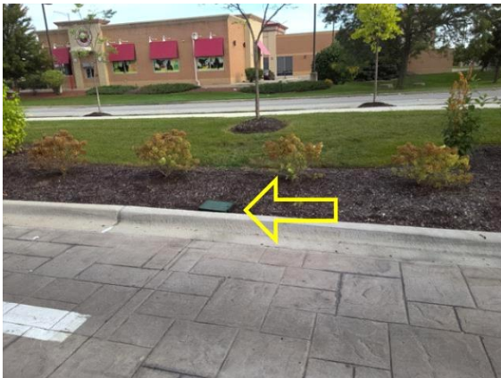
Landscaping/Rodent Traps/Exposed Wires:
