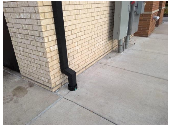
Roof Drainage System Canes:
