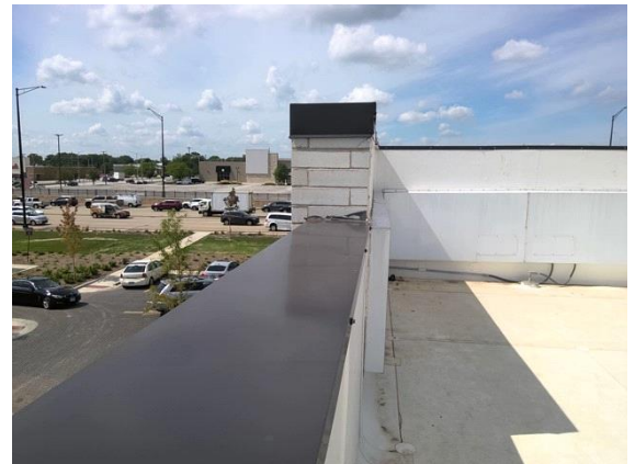
Parapet Wall Panera, Smashburger:
